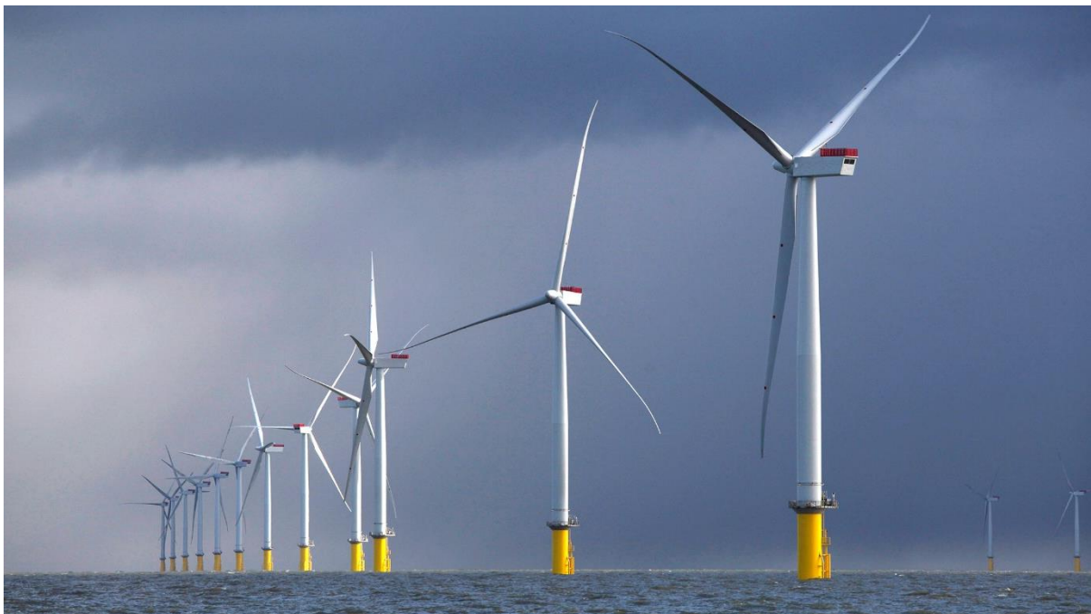
Figure 53: Greater Gabbard Offshore Wind Farm - Operated and Maintained from Lowestoft
