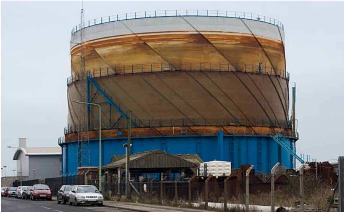
Figure 41: Gasometer (now disused) on Gas Works Road.
