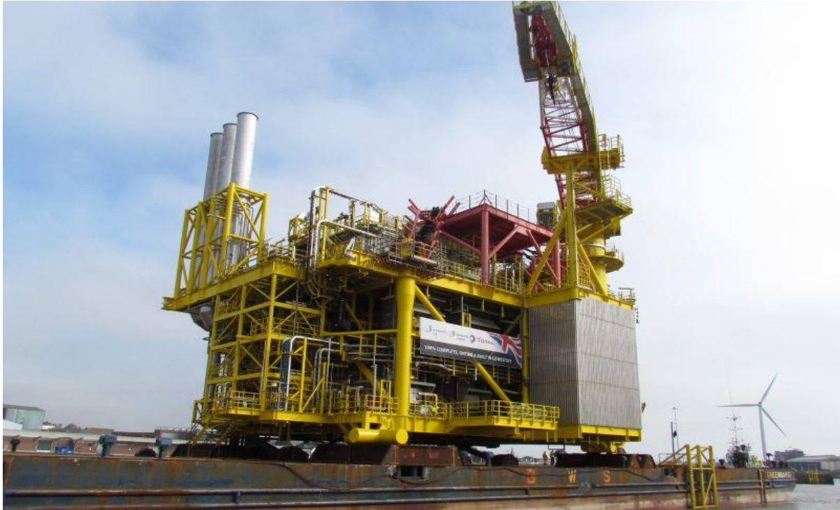
Figure 50: Offshore Power Generation Module, fabricated by Sembmarine SLP for Maerk's Culzean Oil & Gas project.
