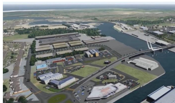
Figure 5: Riverside Road Enterprise Zone area and Jeld-Wen site with artist's impression of the Lake Lothing Third Crossing
