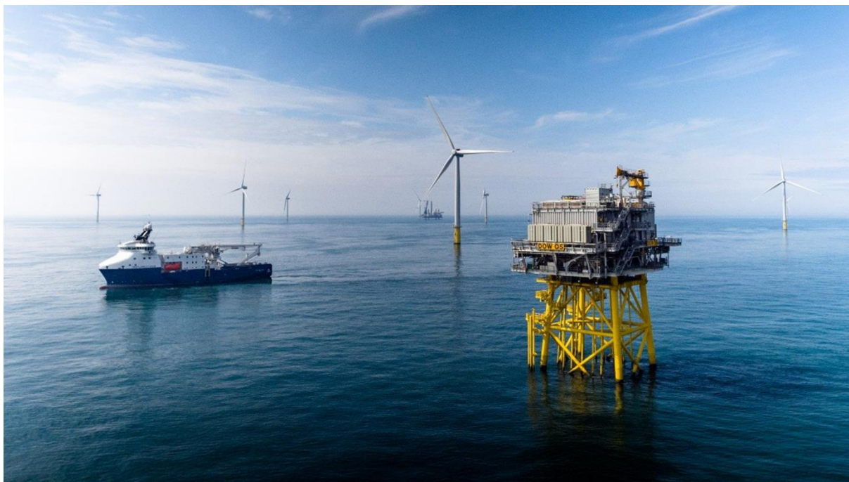
Figure 26: Dudgeon Offshore Wind Farm / Offshore Substation (front right) designed and fabricated at Sembmarine SLP yard in Lowestoft
