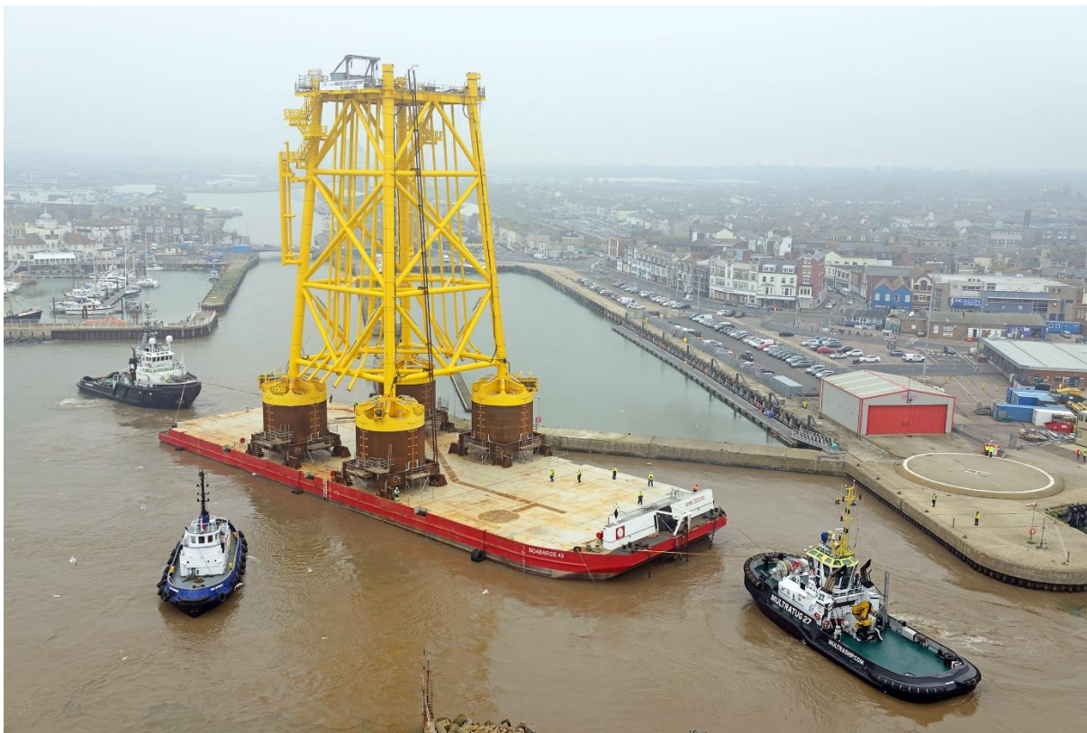
Figure 33: Offshore Wind Substation Foundation being loaded out from Sembmarine SLP Yard
