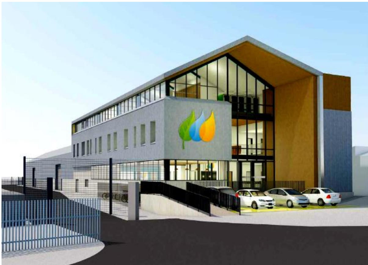
Figure 51: Scottish Power Renewables' East Anglia One Operations Base - currently under construction in Lowestoft
